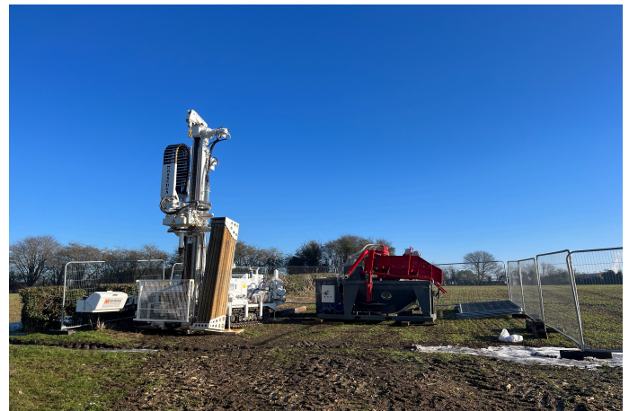
The drilling rig and shaker in position.
